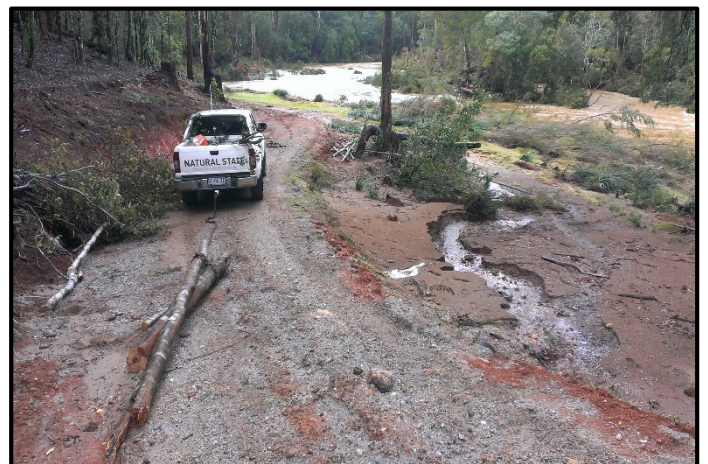
Photo 7: Once the water level drops and the emotions settle, the clean-up begins. The water level was 1m higher than the vehicle.
