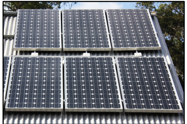
Photos 2&3: Top – Our battery bank which powers our house and business. 48 Volt wired in series with a 6 Kw inverter charger and 240 Volt output. Bottom – Some of our photovoltaic solar panels.
